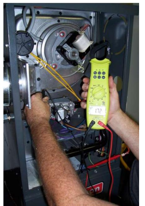
In this example the meter is reading 1.7 micro amps. You need to have >1.0 micro amps for the furnace to continue its cycle. Less than 1.0 micro amp and the furnace will shut down and try to recycle. It will try to recycle 3 times and then go into a 1 hour soft lock out.
