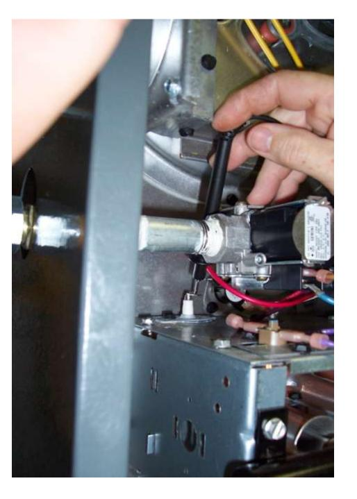
See how many micro amps the meter is reading.
