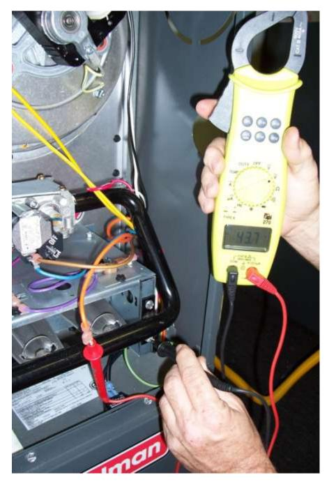
Test to see if there is have voltage going to the flame sensor.
