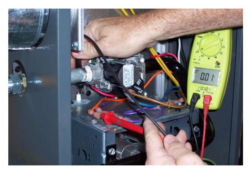
Insert one probe into the female end of the terminal
